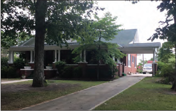
Figure 7.6. Façade, Facing North
