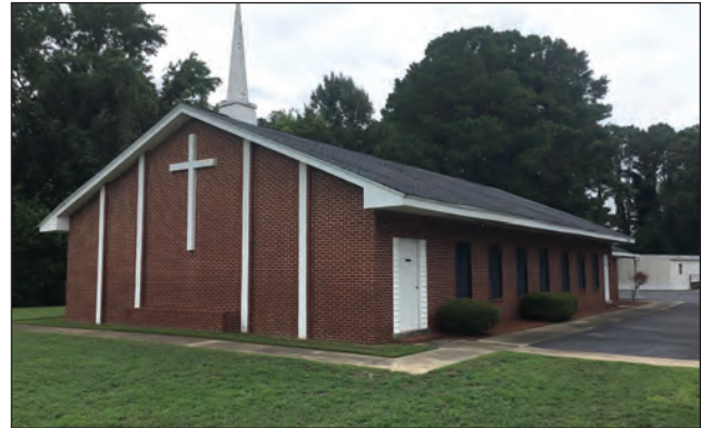
Figure 12.3. Oblique of Southeast Corner, Facing Northwest
