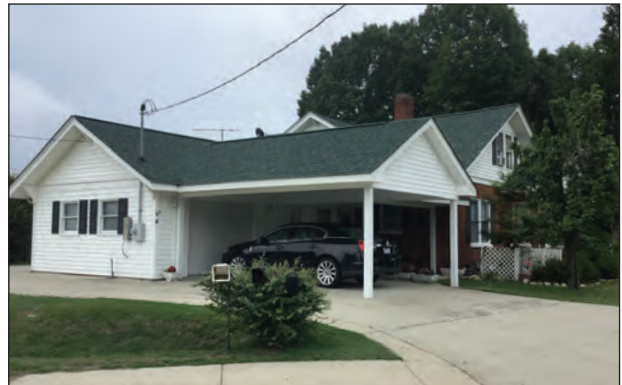
Figure 7.9. Garage Addition, Facing South
