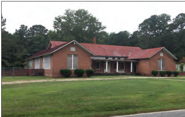
Figure 5.2. Façade Oblique, Facing West
