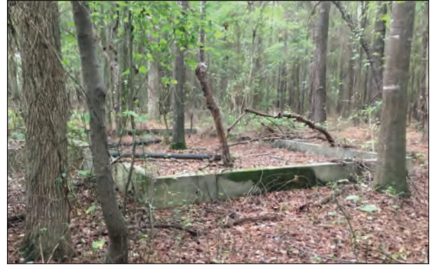
Figure 5.7. Septic Tank, Facing South
