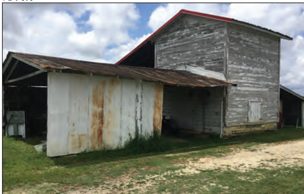
Figure 11.12. Northeast Elevation, Facing Southwest
