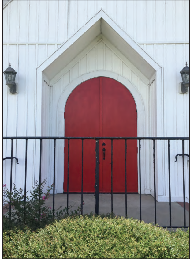
Figure 8.3. Door Detail, Facing South
