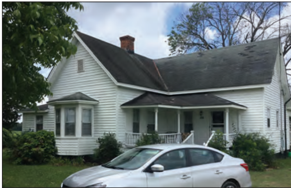
Figure 11.2. Façade Oblique, Facing Southwest
