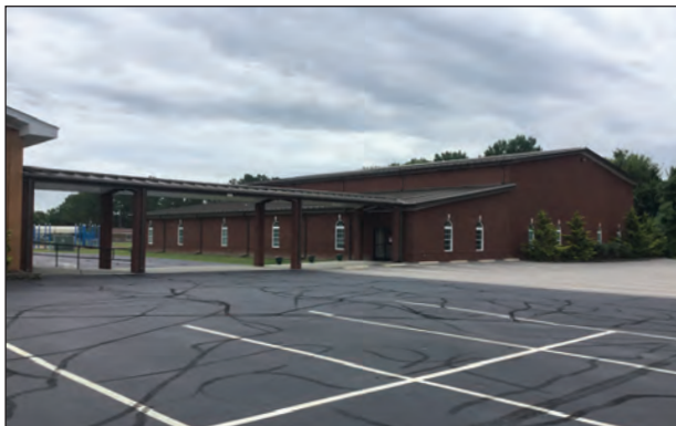
Figure 6.8. Auditorium, Facing Southeast
