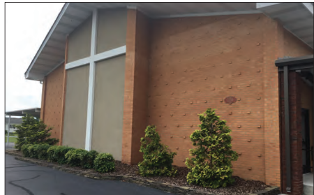
Figure 6.3. Façade View, Showing Brick Work, Facing Northeast
