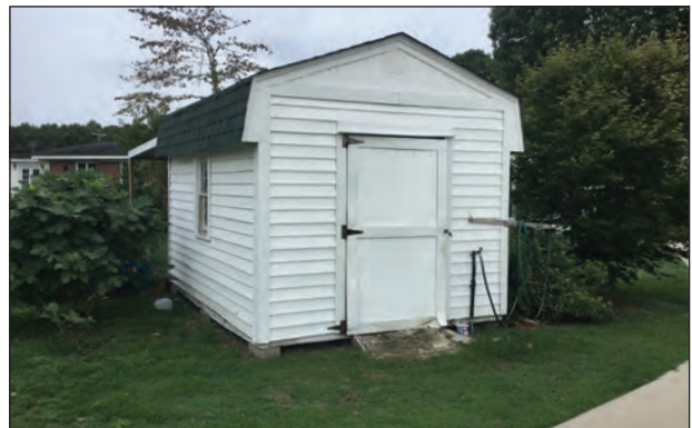
Figure 7.11. Circa 1980 Shed, Facing Southeast
