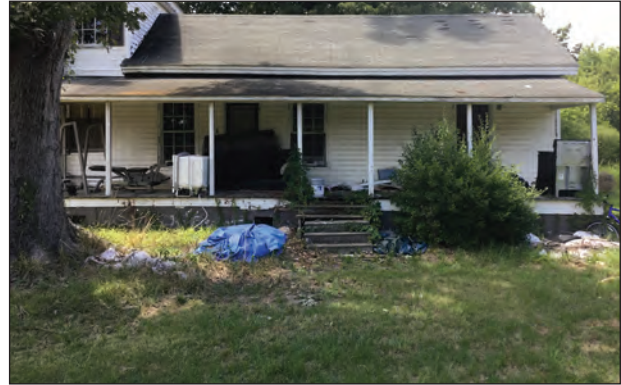
Figure 4.6. Porch on Addition, Facing Northwest
