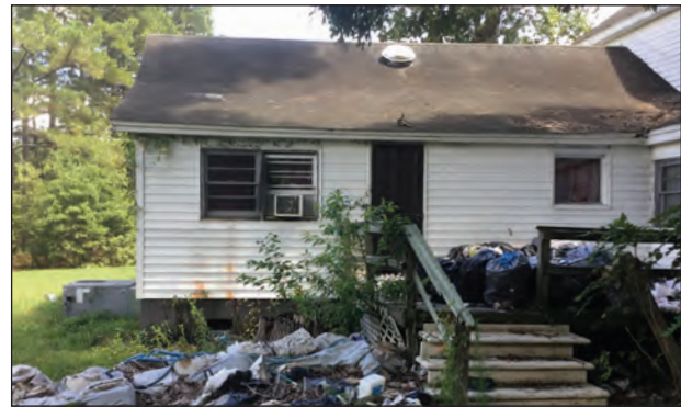
Figure 4.8. Rear Addition, Facing Southeast
