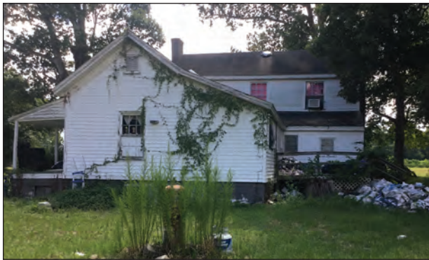
Figure 4.7. Northeast (Rear) Elevation, Facing Southwest
