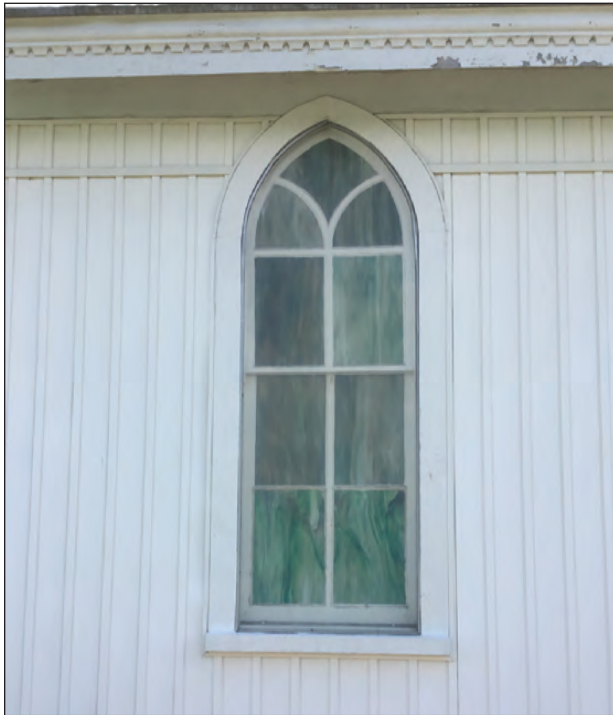
Figure 8.4. Window Detail, Facing Southeast
