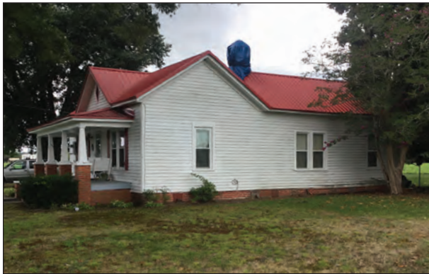
Figure 10.4. Northeast Elevation, Facing Southwest
