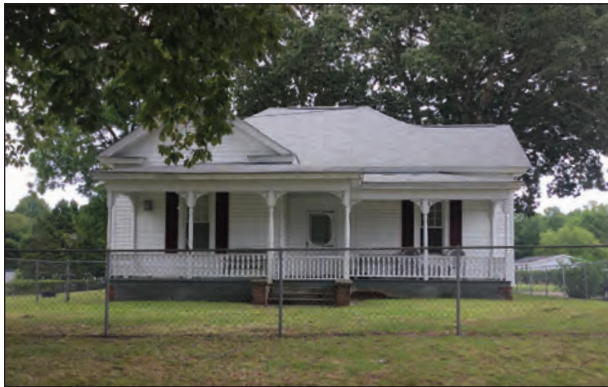
Figure 9.2. Façade, Facing East
