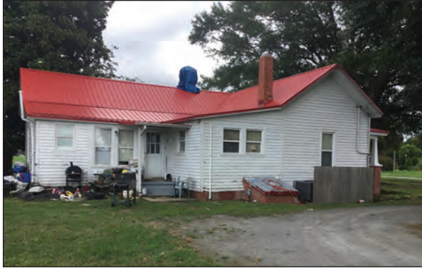
Figure 10.6. Rear Porch Oblique, Facing East
