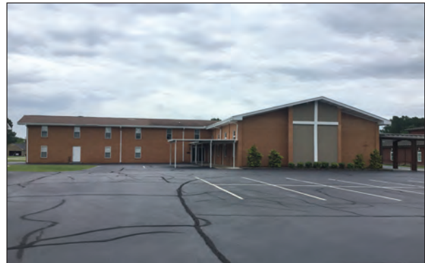
Figure 6.5. West Elevation, Facing South
