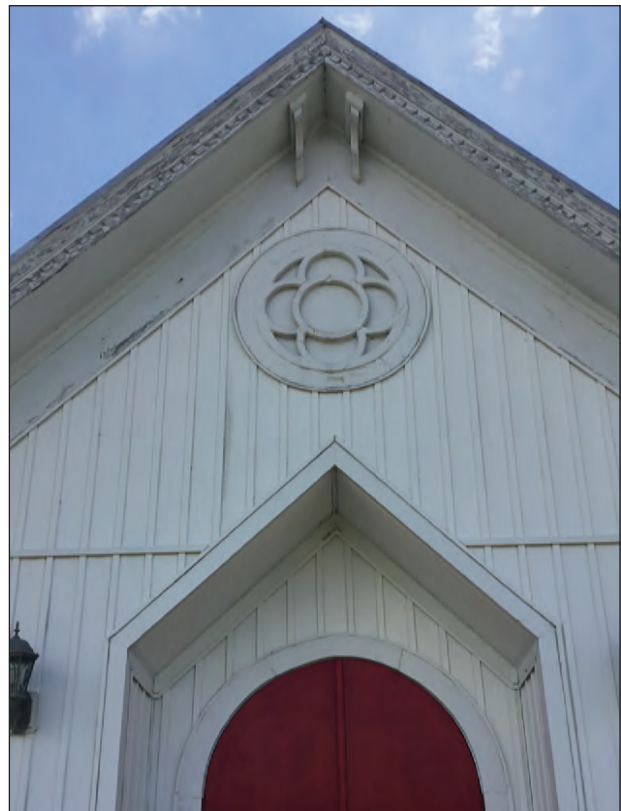
Figure 8.6. Rosette Detail, Facing South
