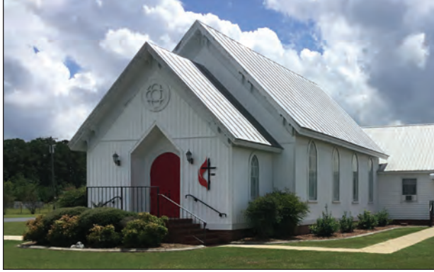
Figure 8.2. Façade, Facing South
