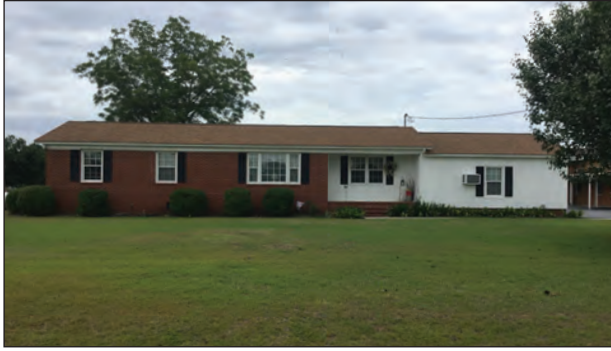
Figure 6.10. Façade of Parsonage, Facing East
