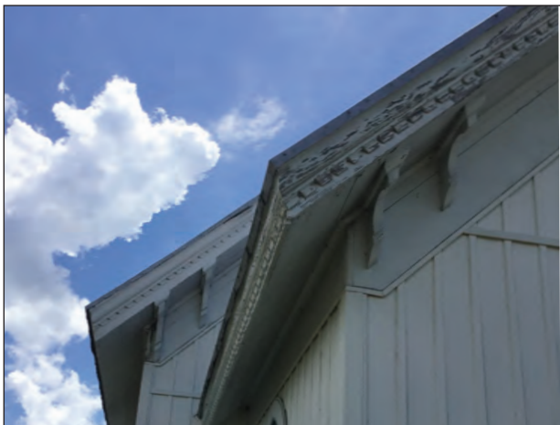
Figure 8.5. Eave Work, Facing South
