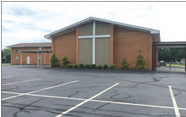
Figure 6.2. 1968 Church Building, Facing East
