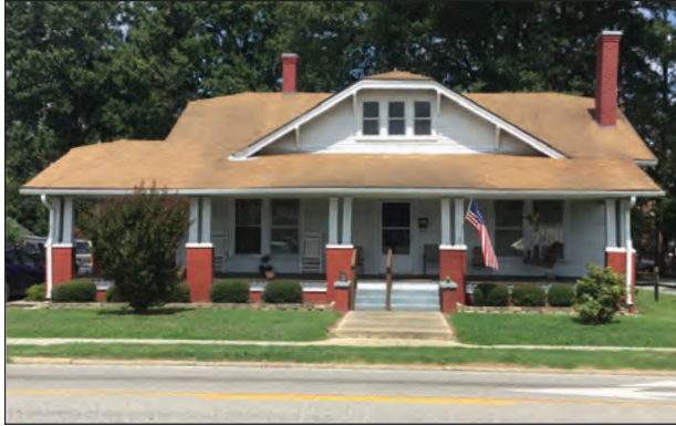
Figure 7.14. Selma Baptist Parsonage (JT0150), Selma, Johnston County
