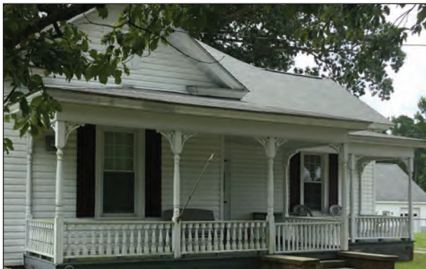
Figure 9.6 Porch Detail, Facing Southeast
