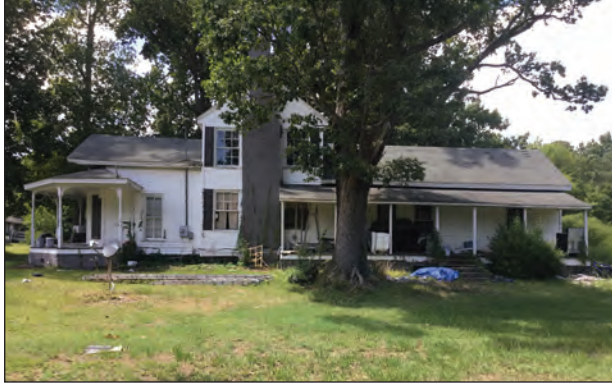
Figure 4.5. Southeast Elevation, Facing Northwest
