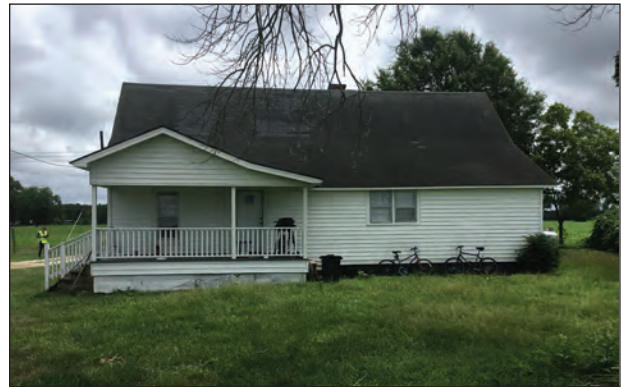
Figure 11.9. West Elevation, Facing East
