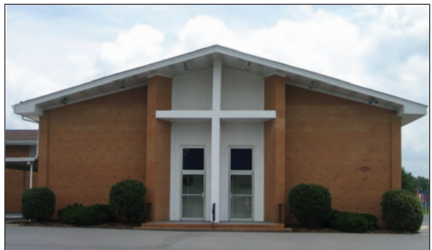
Figure 6.16. Grace Baptist Church, Pre-Renovation
