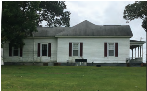
Figure 9.5. North Elevation, Facing South
