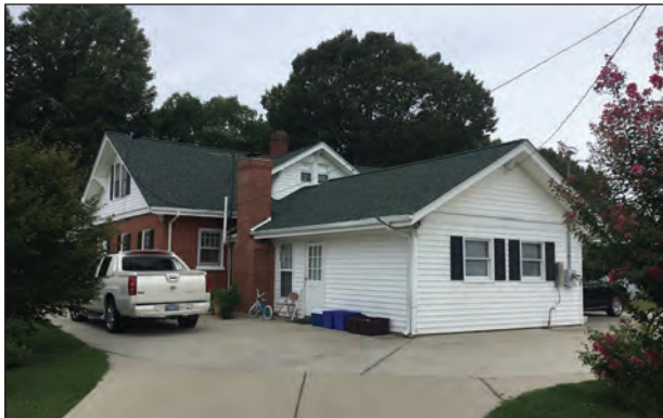
Figure 7.8. Garage Addition, Facing West
