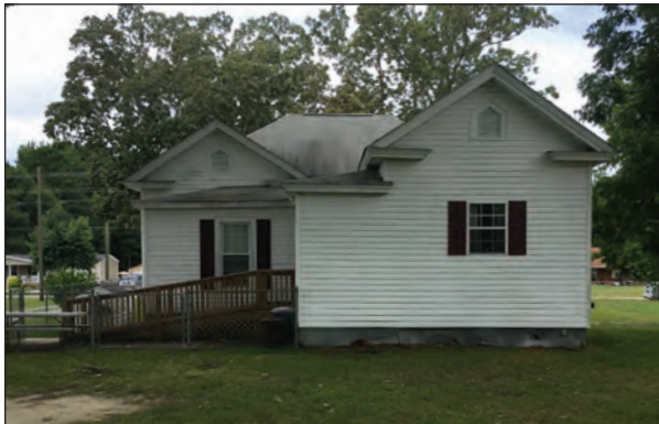
Figure 9.4. Rear Elevation, Facing West
