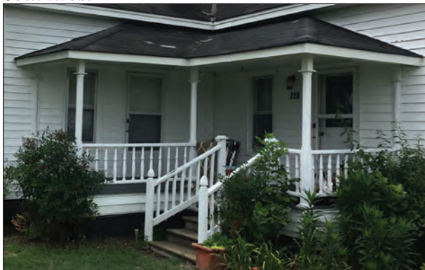
Figure 11.4. Porch Detail, Facing Southwest
