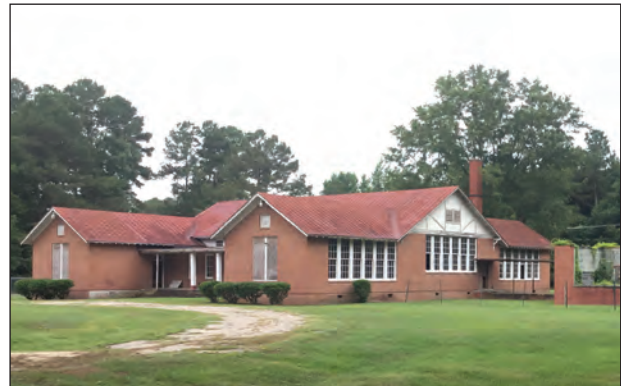
Figure 5.3. Façade Oblique, Facing Southeast
