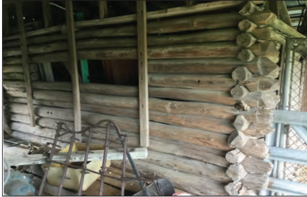
Figure 11.14. Log Pen in Interior of Pole Barn, Facing Northeast
