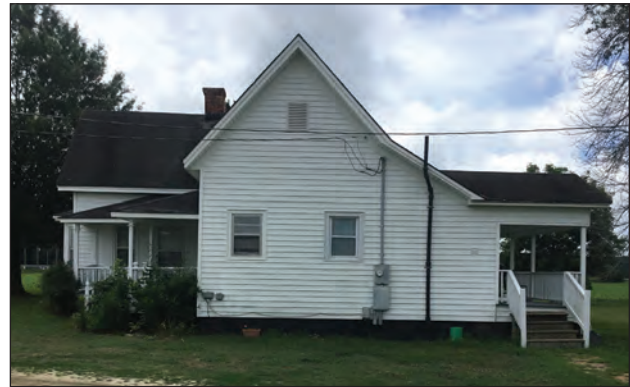
Figure 11.3. North Elevation, Facing South
