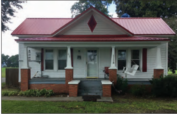
Figure 10.2. Façade, Facing Northwest
