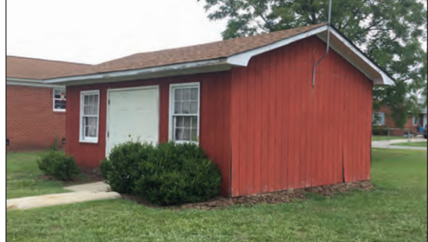
Figure 6.11. Shed, Facing Northwest
