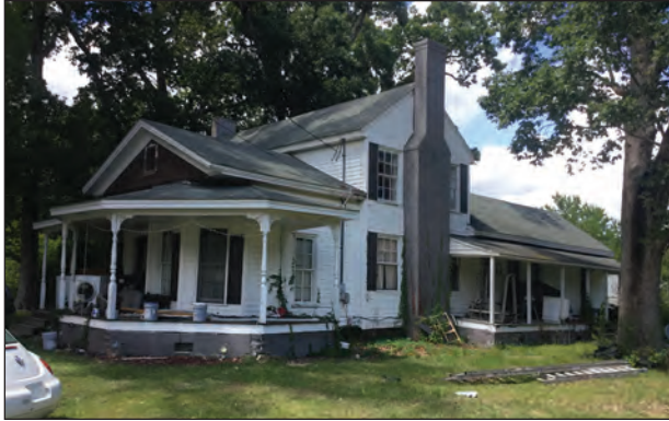
Figure 4.2. Oblique View, Facing North
