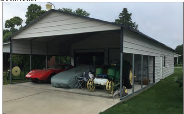
Figure 7.13. 1990 Garage, Facing South
