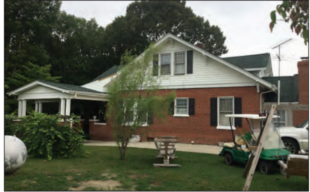
Figure 7.7. Southeast Elevation, Facing Northwest
