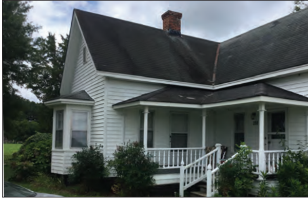
Figure 11.6. East Facing Addition, Facing Southwest
